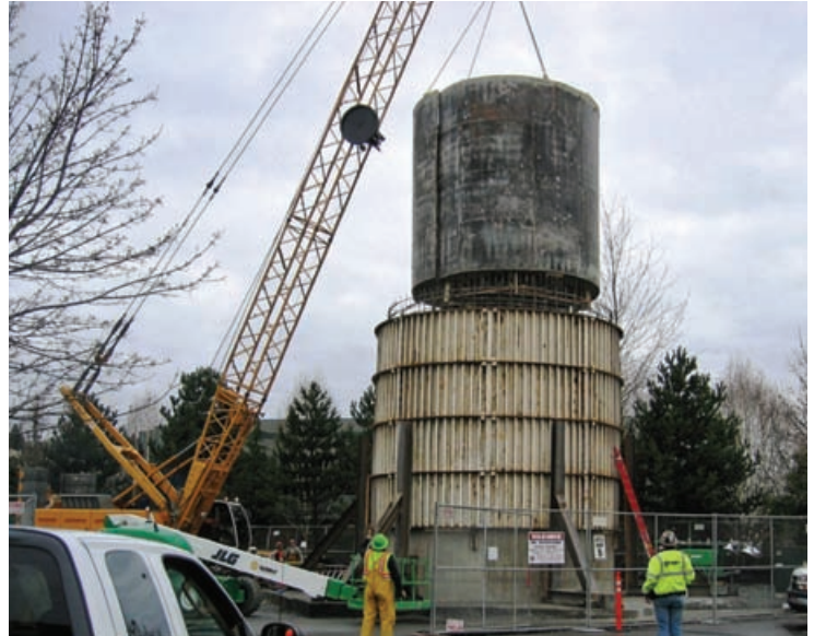
Sunken caisson for the microtunnel receiving pit, North Creek Connector.
